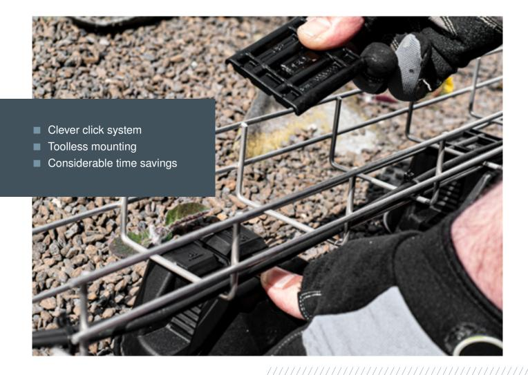
Provides the decisive installation benefits for the mounting of GR-Magic® mesh cable trays on flat roofs quickly and simply: the plug-in mesh cable tray adapter for the 165 MBG roof conductor holder.
